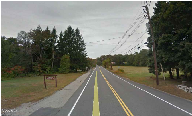
EXISTING SECTION HAYDEN ROWE STREET (SR85) COLLEGE STREET TO GRANITE STREET LOOKING NORTH
