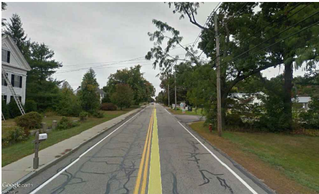
EXISTING SECTION HAYDEN ROWE STREET (SR85) CHESTNUT STREET TO EMC FIELD LOOKING NORTH
